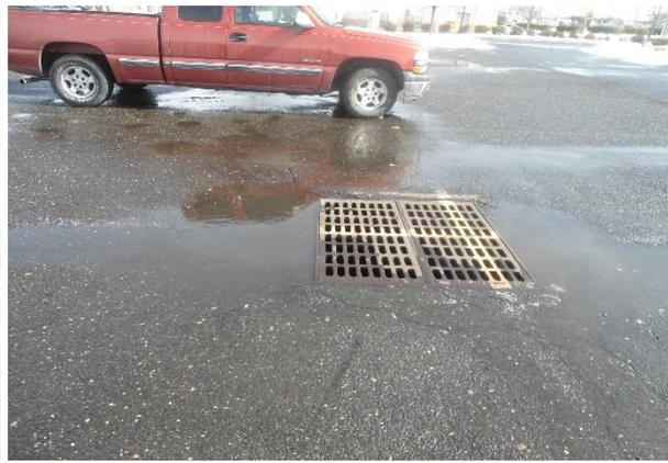
Parking spaces could be repaved with pervious pavement to intercept runoff prior to storm drains, thereby reducing loads to storm sewers. Bioretention systems could also be utilized to collect runoff. A preliminary soil assessment for this site suggests that the site's existing soils have suitable drainage characteristics for green infrastructure.
